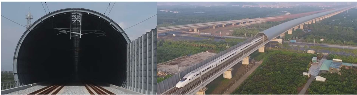
Figure 2: Shenzhen-Maoming Guideway Enclosure
