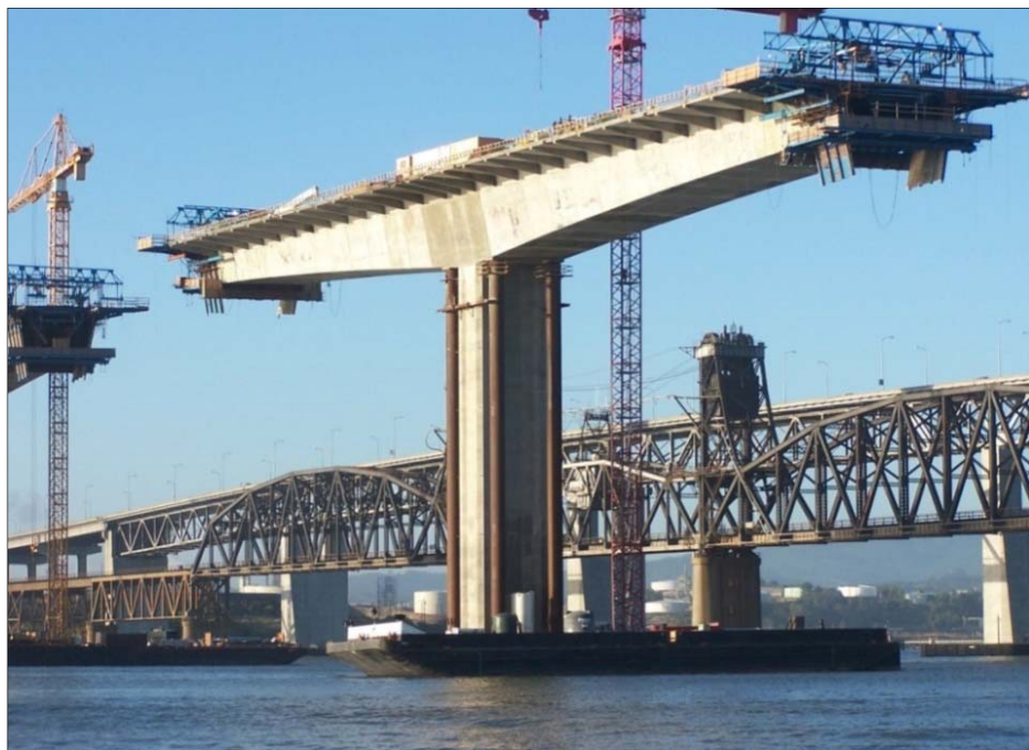
Figure 4-9 Form Travelers and Temporary Supports in Balanced Cantilever Construction
