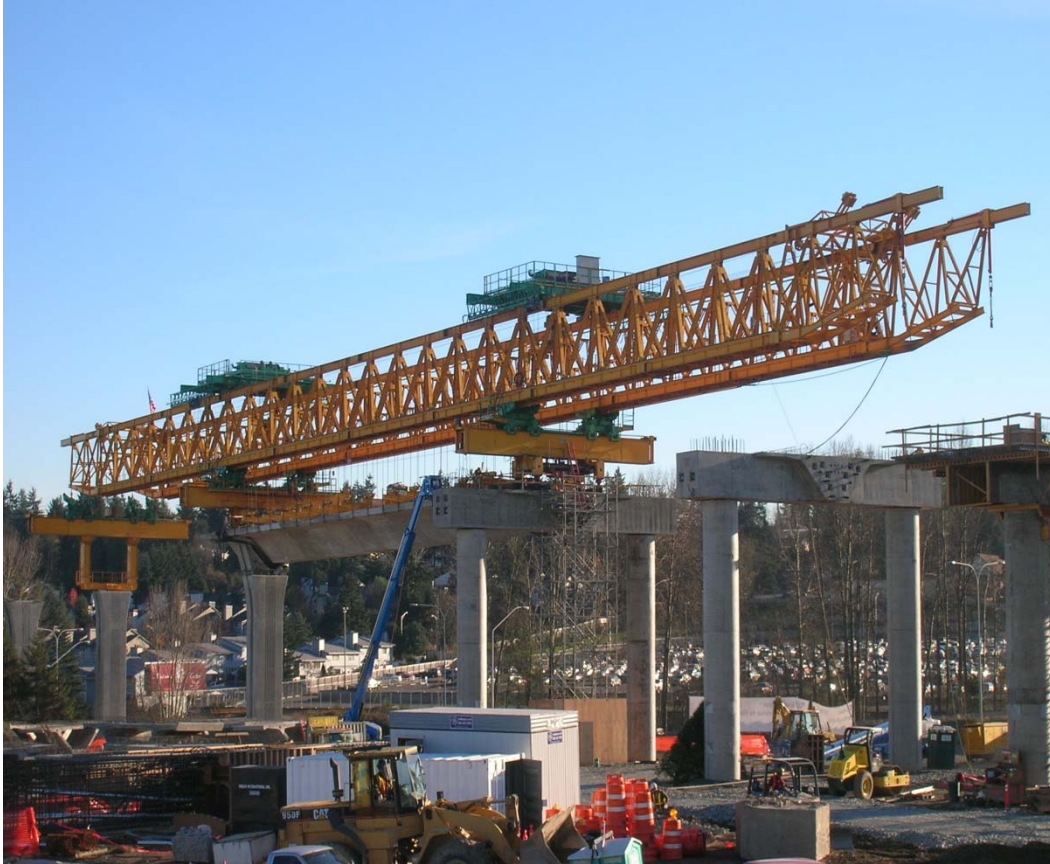
Figure 4-6 Precast Segmental Construction
