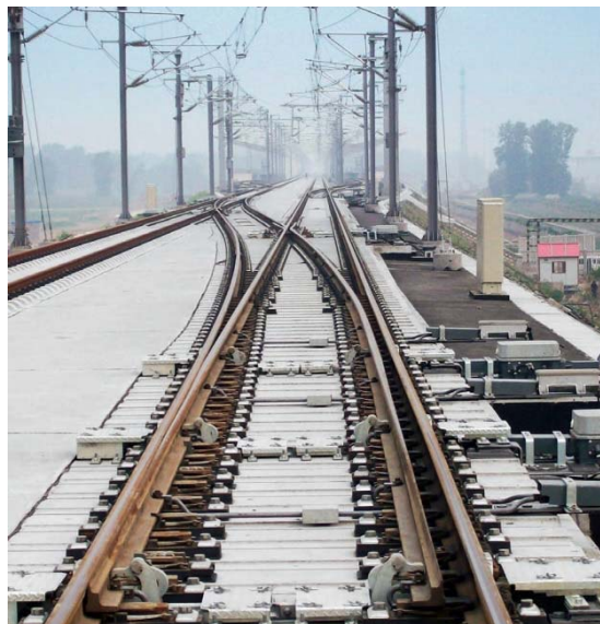
Figure 4-17 Track Turnouts - China HSR
