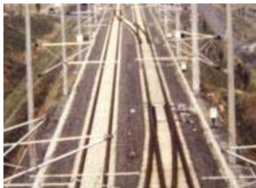
Figure 4-14 Ballast Track with Mats - Japan
