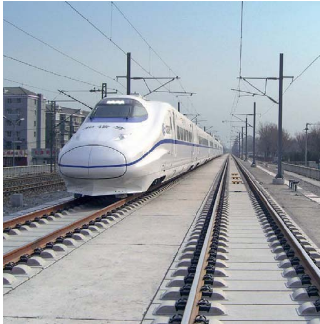
Figure 4-16 Slab Track - China HSR
