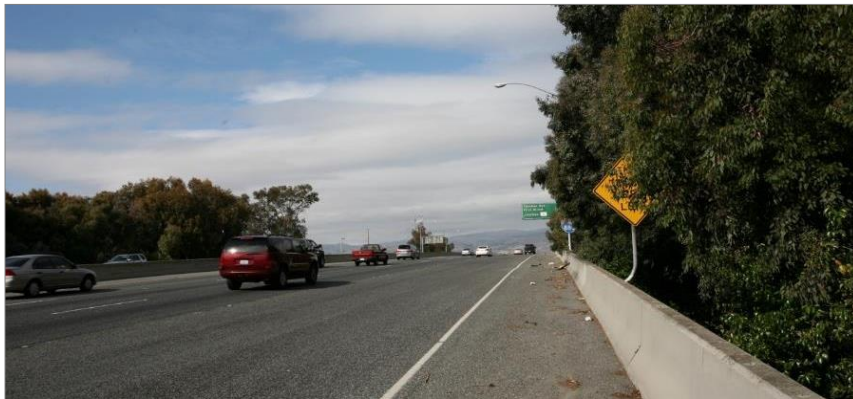
KVP 2—Existing Conditions
