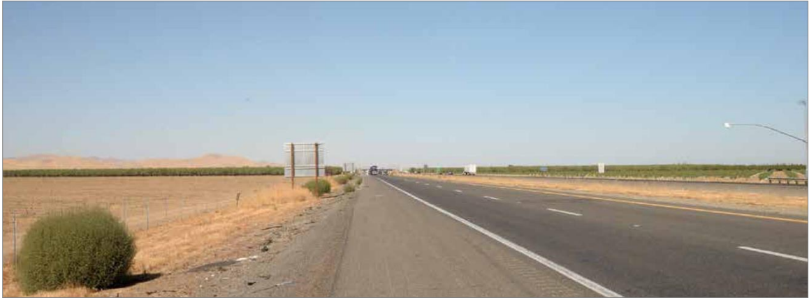
KVP 33—Existing Conditions
