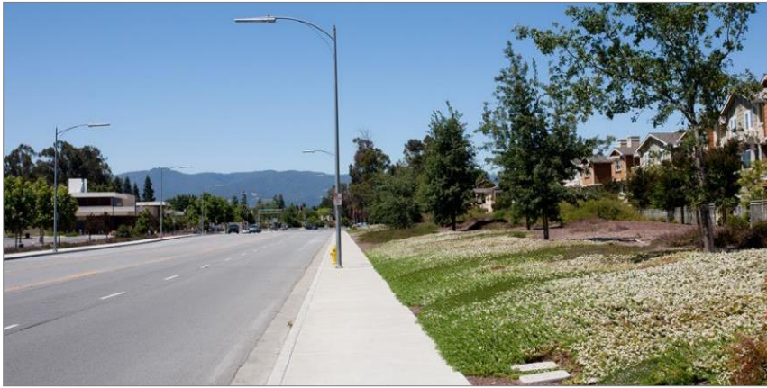
KVP 13—Existing Conditions
