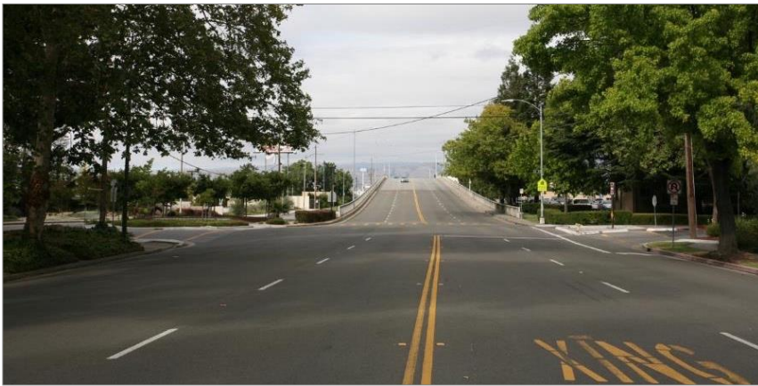
KVP 3—Existing Conditions
