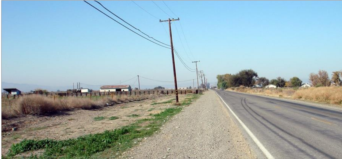
KVP 35—Existing Conditions
