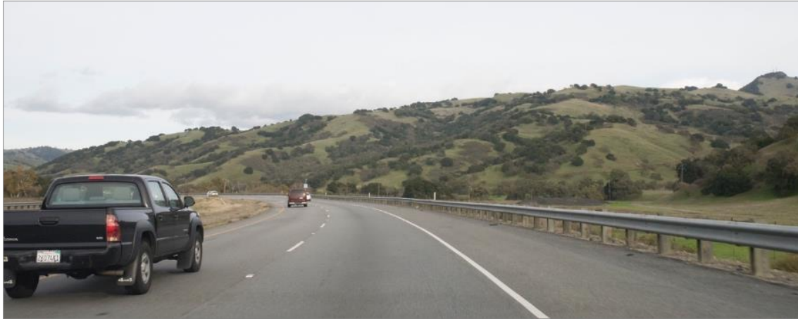
KVP 30—Existing Conditions
