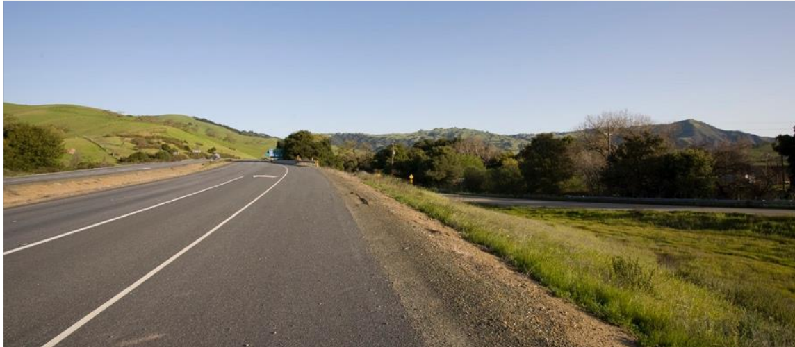
KVP 28—Existing Conditions
