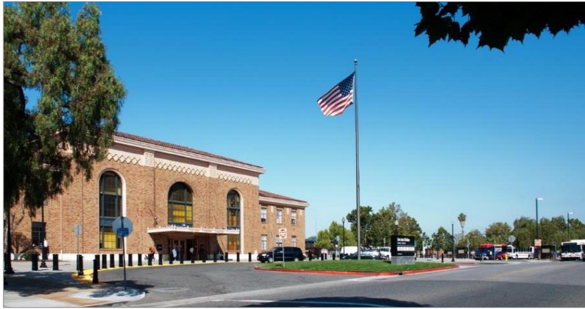
KVP 6—Existing Conditions
