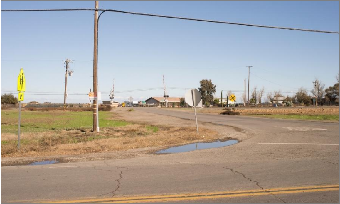
KVP 34—Existing Conditions
