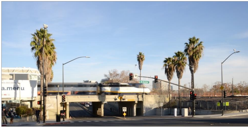
KVP 4—Existing Conditions
