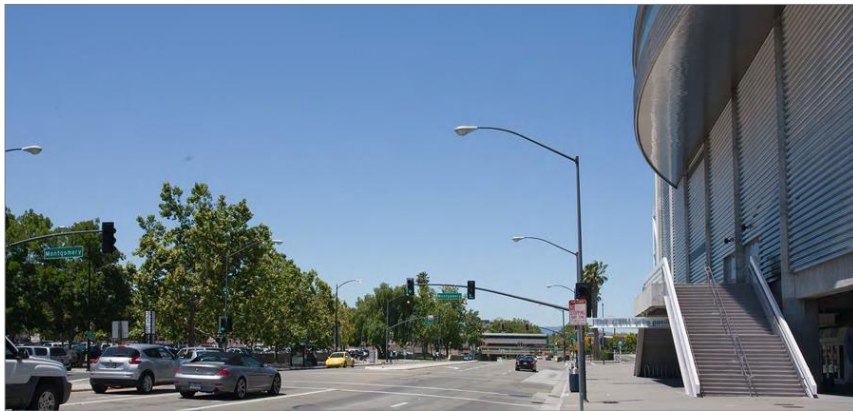
KVP 5—Existing Conditions
