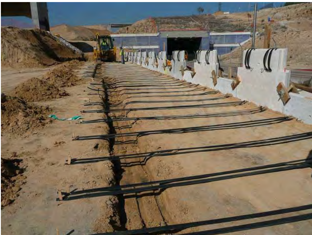
Figure 4. Reinforced earth wall execution
