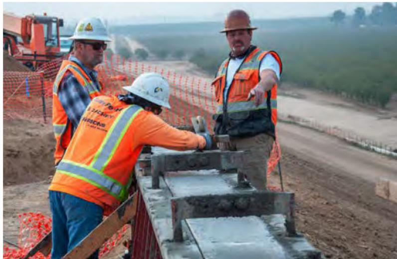
PHOTO: AVENUE 11 GRADE SEPARATION PROJECT WILL CARRY TRAFFIC OVER BNSF TRACKS AND FUTURE HIGH-SPEED RAIL LINES.
