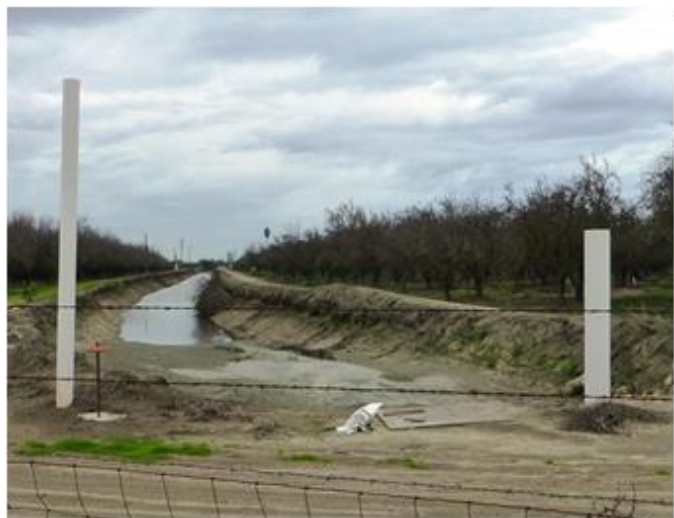
Camera facing south from SR 152 Photo taken 12/19/2014
