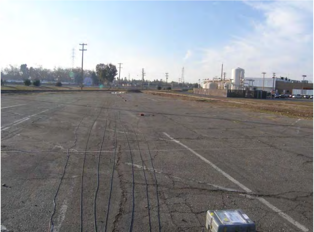
VIBRATION MEASUREMENT SITE V1
