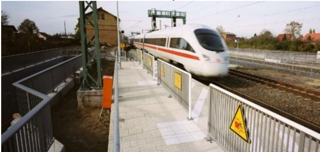
Figure 3.5.5: Additional Deutsch Bahn Platform Safety Measures
