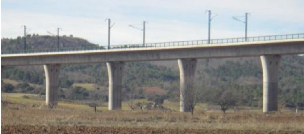
Spain HSR Aerial Structure
