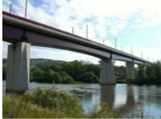
Steel Girder, Mosel, Germany
