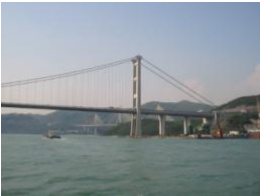
Cable Suspension, Hong Kong
