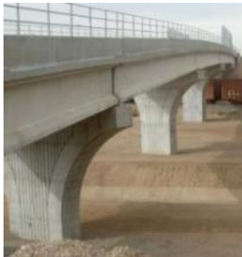
Phoenix Light Rail
