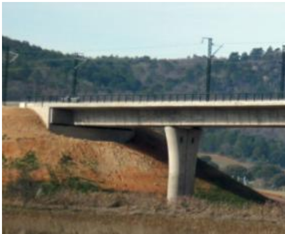
Natural Abutment, Spain HSR
