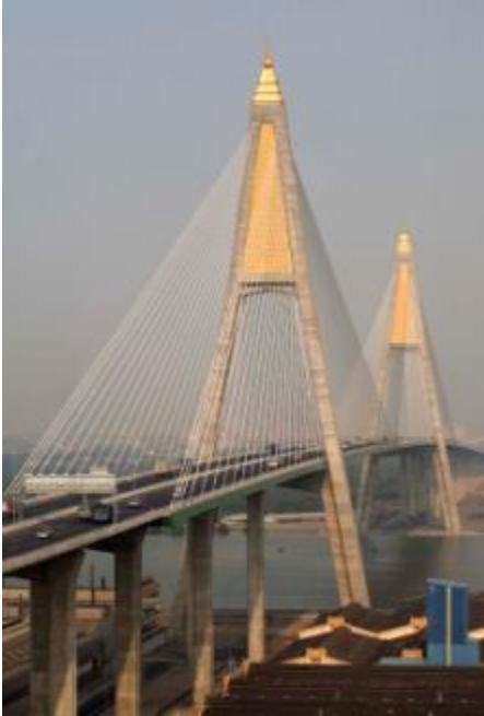
Kanchanapisek Bridge Thailand
