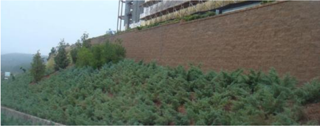
Effective Reduction of Apparent Wall Height
