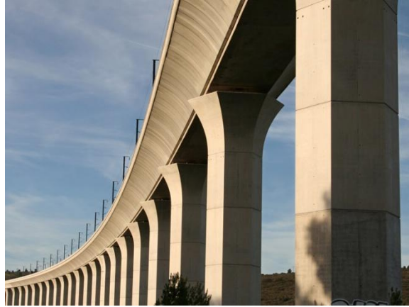
France HSR Box Girder
