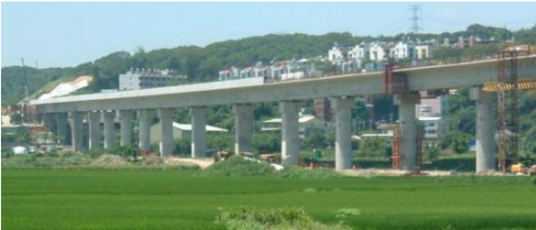
Taiwan HSR Aerial Structure
