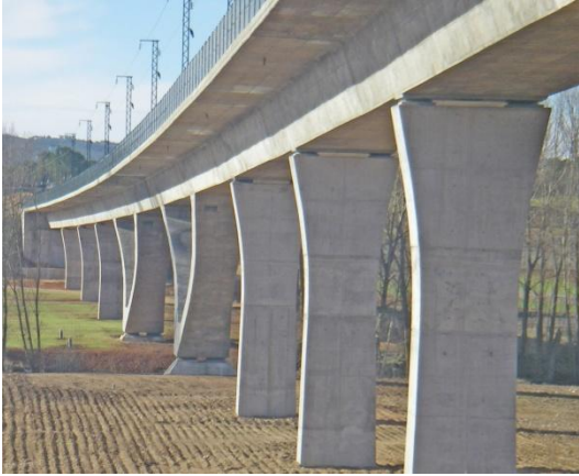
Spain HSR Box Girder
