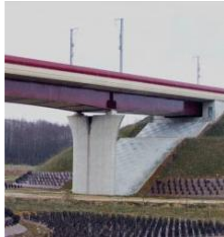
Retained Abutment, France HSR
