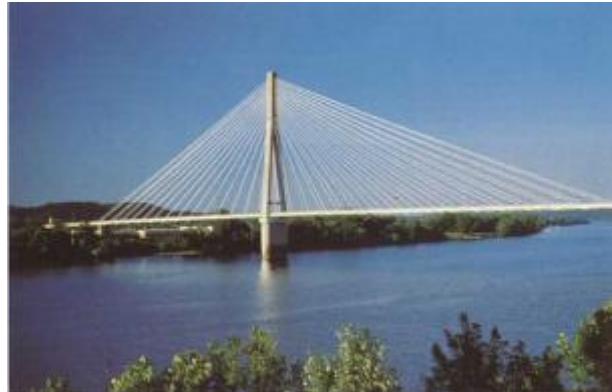
Cable Stayed, East Huntington
