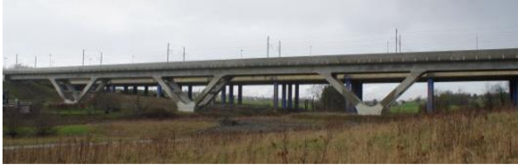
Multiple columns: Ruyff Valley Aerial Structure, Belgian HSR
