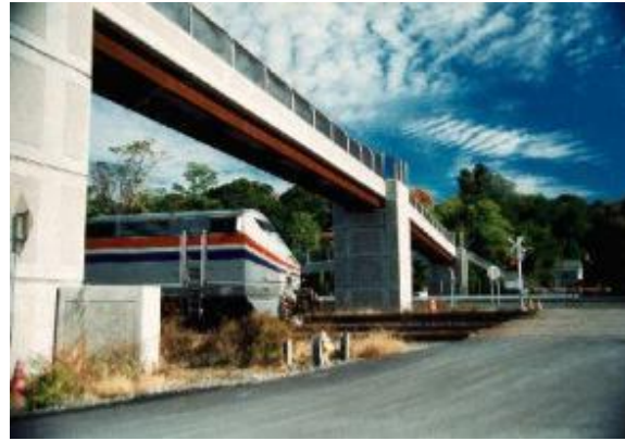
Functional: Route 9, MTA New York
