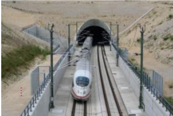
Low Maintenance: German HSR Portal
