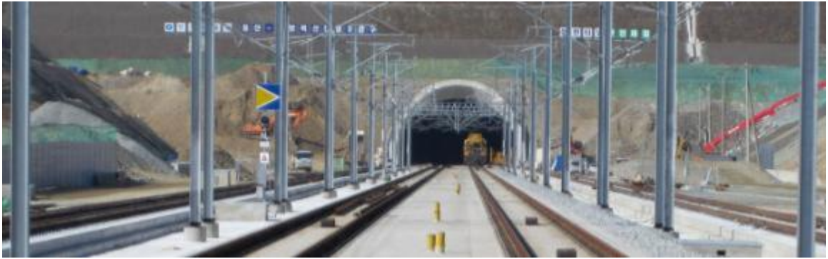
Korea HSR Tunnel Portal
