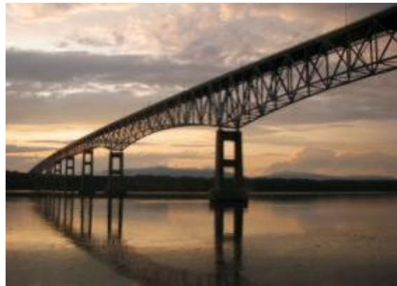
Steel Truss, New York
