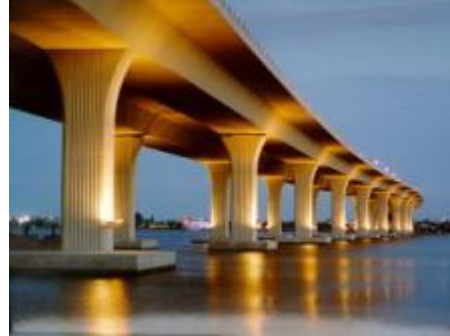
Roosevelt Bridge, Stuart, Florida
