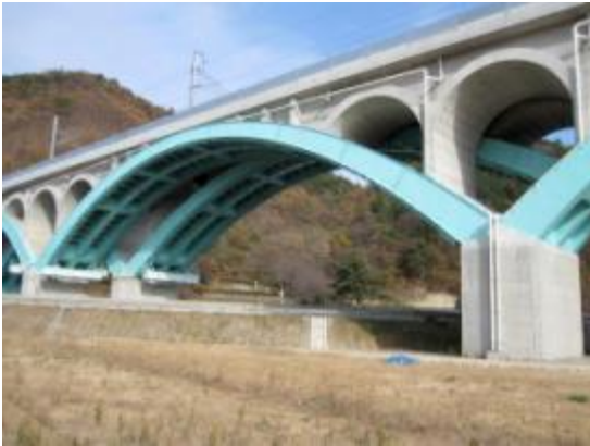
Steel Arch, Korea HSR
