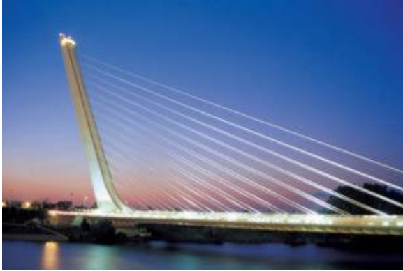
Alamillo Bridge, Spain
