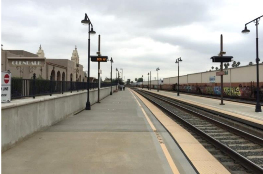
Existing view from the Glendale Transportation Center in the city of Los Angeles, looking southeast.
