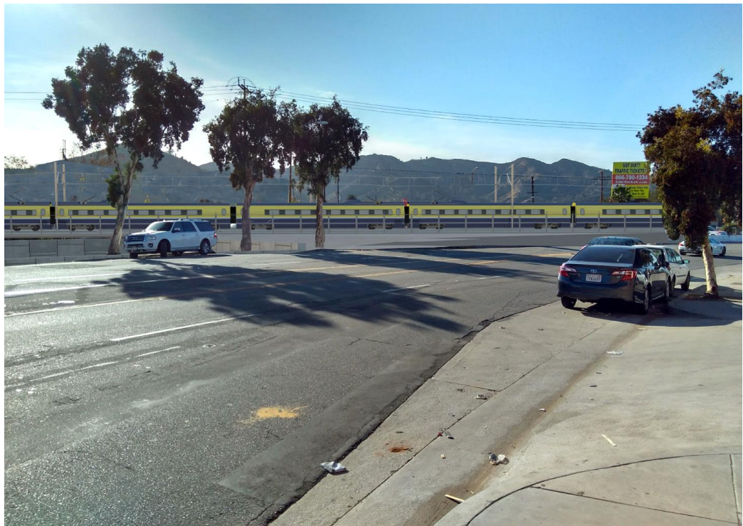
Simulated view of the High-Speed Rail Build Alternative from San Fernando Road in the city of Los Angeles, looking east.
