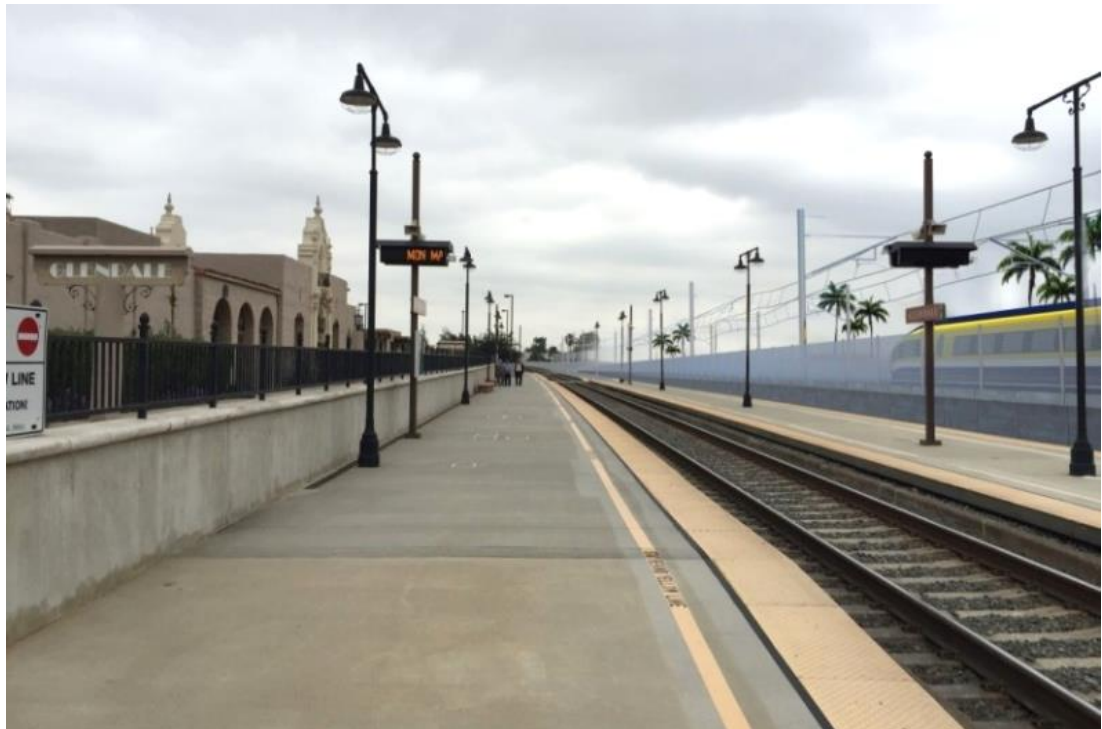
Simulated view of the High-Speed Rail Build Alternative from the Glendale Transportation Center in the city of Los Angeles, looking southeast.
