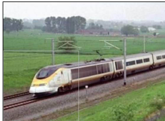
Figure 2-2 Example of an At-Grade Profile Showing Contact Wire System and Vertical Arms of the Pantograph Power Pickups
