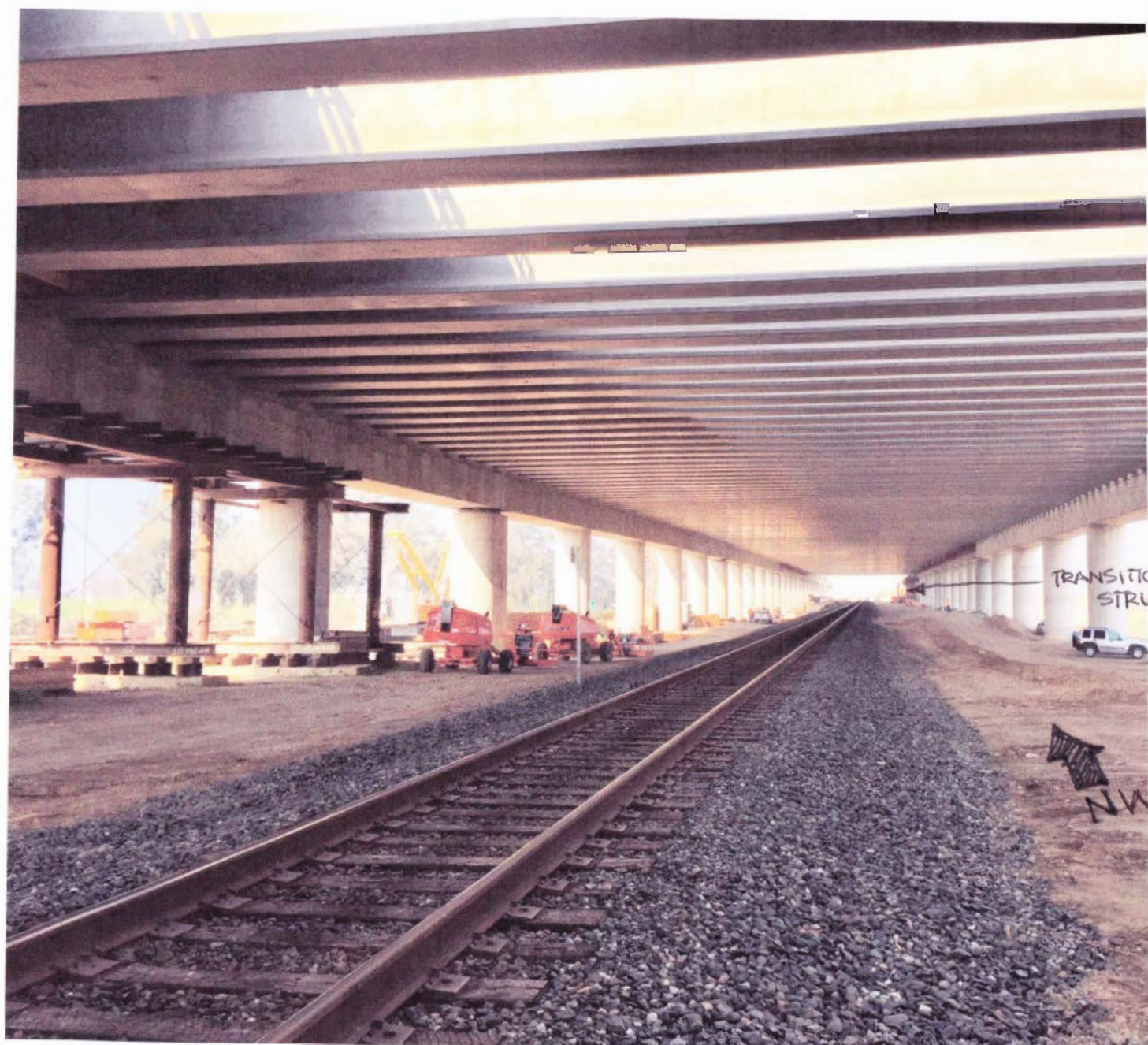
HSR STRUCTURE OVER UPRR TRACKS NEAR HERNDON DRIVE, LOOKING NORTHWEST
