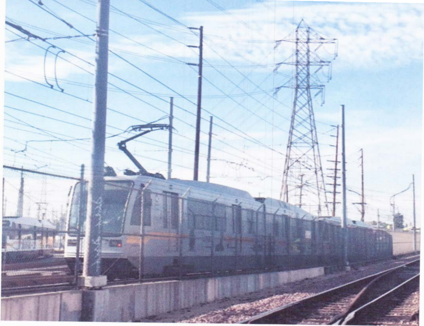
ATTACHMENT 8 METRO GREEN LINE UNDER HIGH VOLTAGE TOWERS
