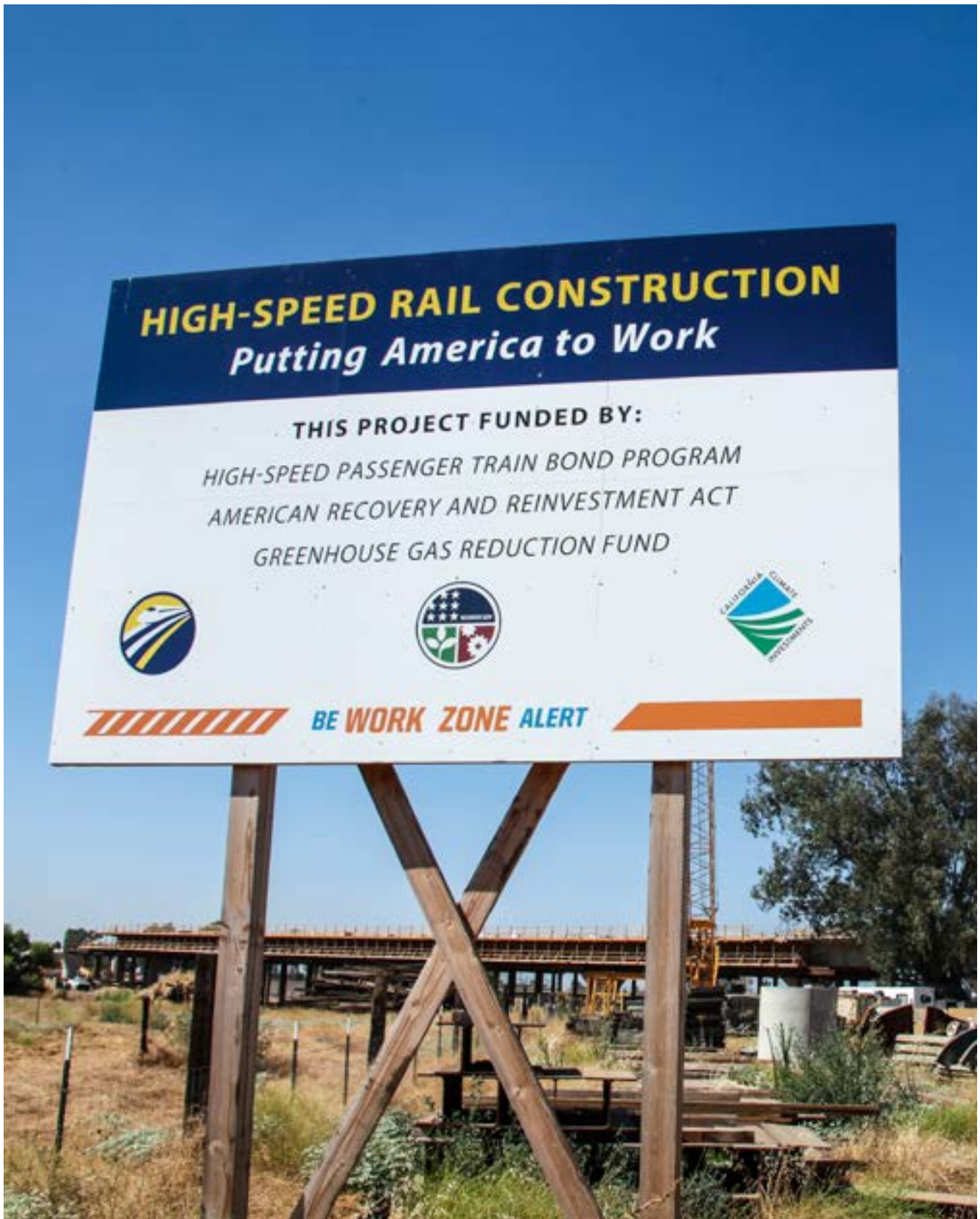
PHOTO: CONSTRUCTION CONTINUES IN THE CENTRAL VALLEY, LAYING THE FOUNDATION FOR THE SYSTEM.
