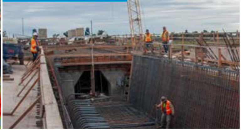
CP 1 SAN JOAQUIN RIVER VIADUCT
