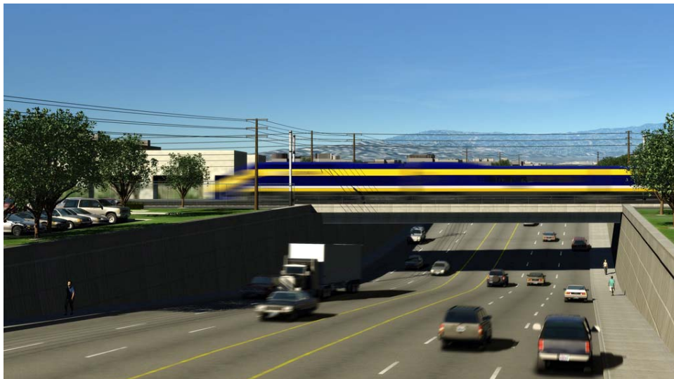
Figure 2.3 A simulation of a grade-separated intersection with the high-speed train passing overhead
