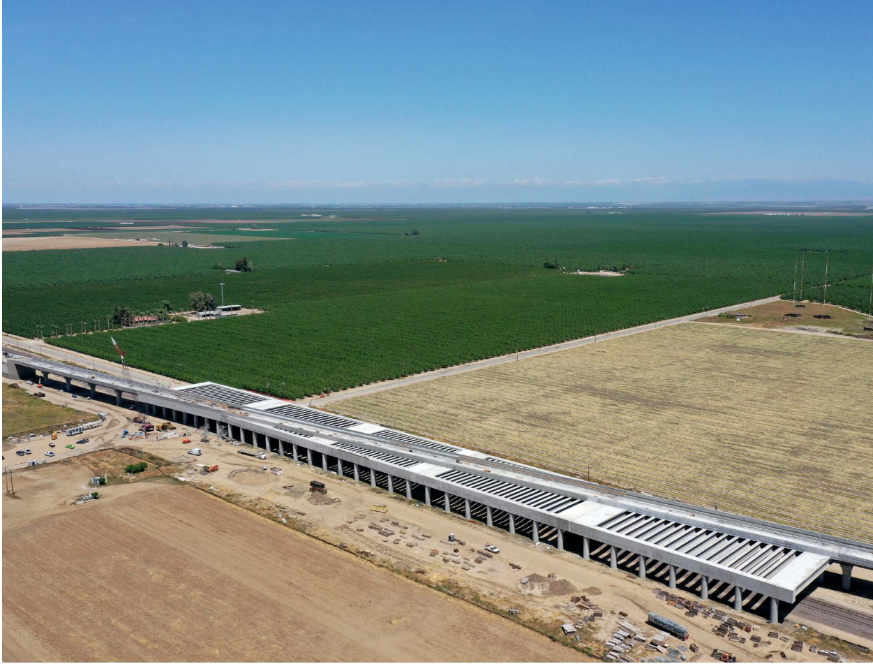
Photo: Wasco Viaduct in Kern County
