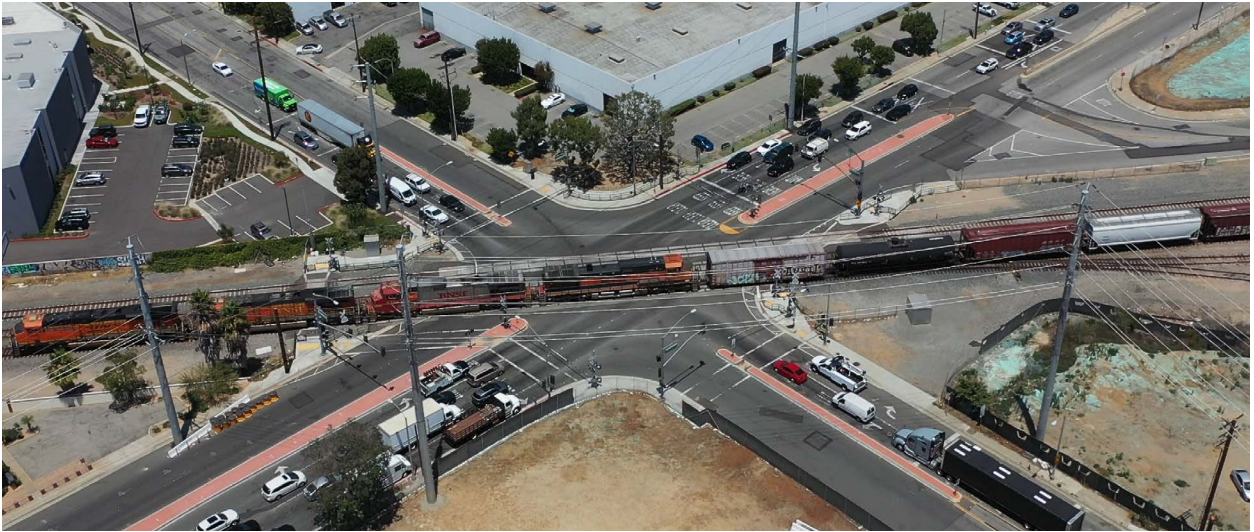
Photo: Rosecrans Avenue and Marquardt Avenue grade separation (before)
