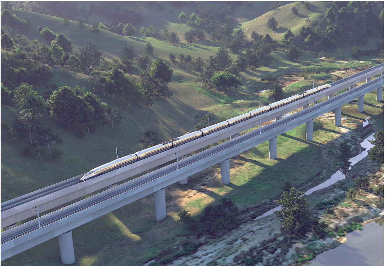
Rendering: High-speed rail will move through the Pacheco Pass area between San José and Merced
