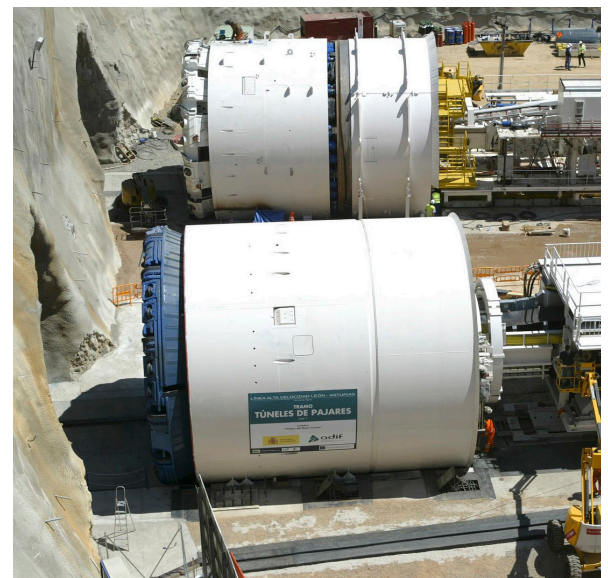
Figure 2. Photo of tunnel boring machines constructing a dual-bore tunnel.
