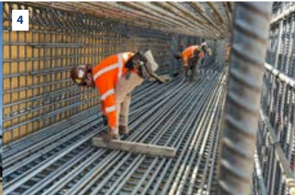
3. & 4. Construction crews installed falsework for edge beams of the Cedar Viaduct located west of State Route 43 in Fresno County. In August, they poured more than 500 cubic yards of concrete in 12 hours.
