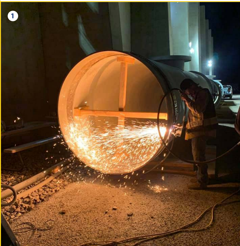
1. & 2. Last February, crews from Dean's Certified Welding descended on two remote pumping stations for the Metropolitan Water District of Southern California, the largest supplier of treated water in the U.S. They were tasked with replacing 72-inch steel pipe segments that go underground and tie into the pumping plant.
