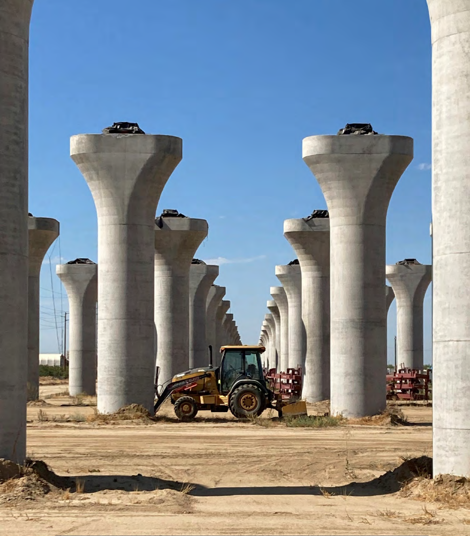
Photo: Future Kings/Tulare station trackway viaduct structure.
