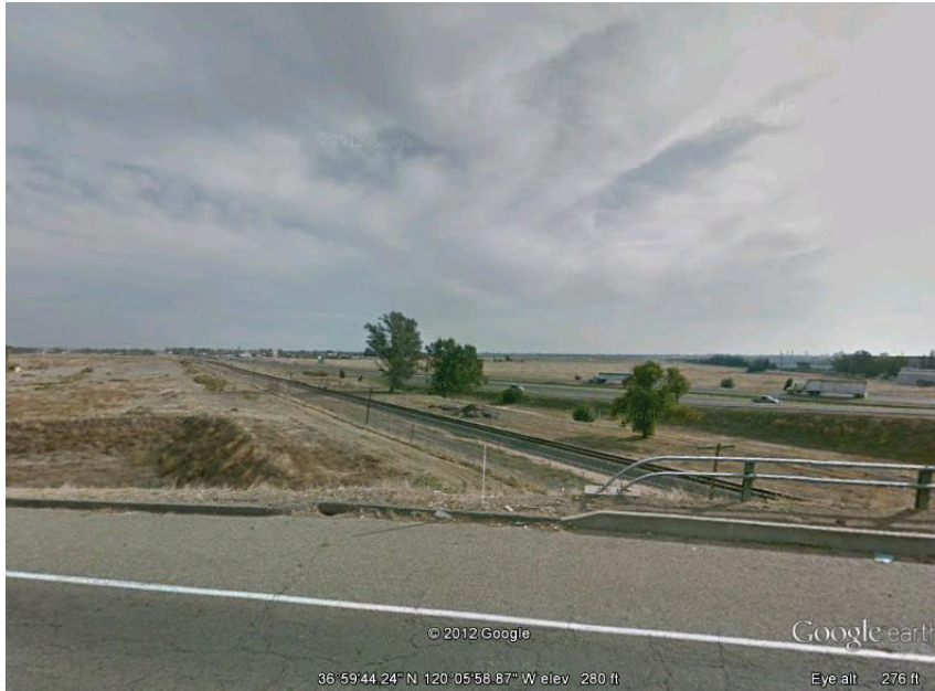
Location 14. Looking south along the elevated UPRR/SR 99 Alternative from Ave 17/SR 99 interchange in the City of Madera. Existing land use is vacant and future land uses are commercial.
