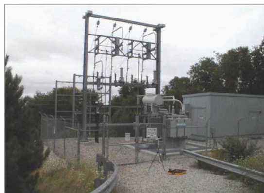
Figure 2-17 Paralleling Station
