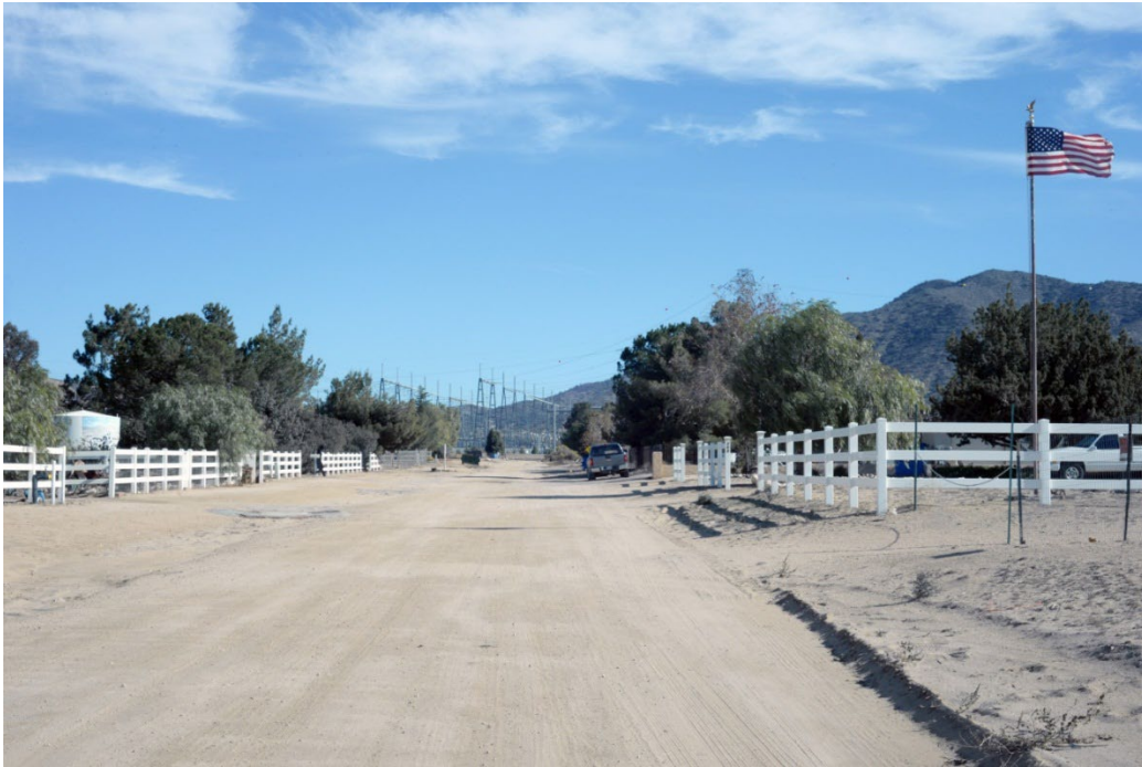
a. Existing View: View to the east along Foreston Drive. The viewpoint is from a dirt road within an isolated neighborhood. Electrical towers and lines associated with the Vincent Substation are visible, creating a distinctly industrial feature in the otherwise rural setting. The view offers moderate visual quality to residents and travelers.
