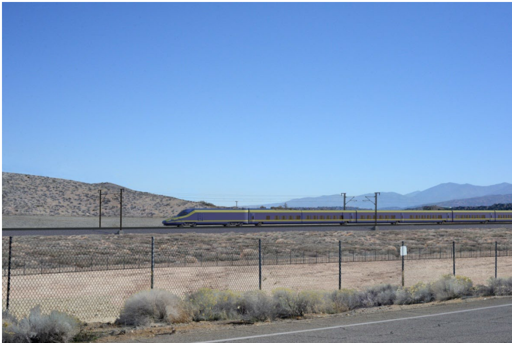
b. Simulated View (Refined SR14, E1, and E2 Build Alternatives): The project would replace Una Lake and its surrounding vegetation with at-grade tracks. Project features would substantially diminish the natural harmony of the existing visual character and have an overall adverse degree of change to visual quality.
