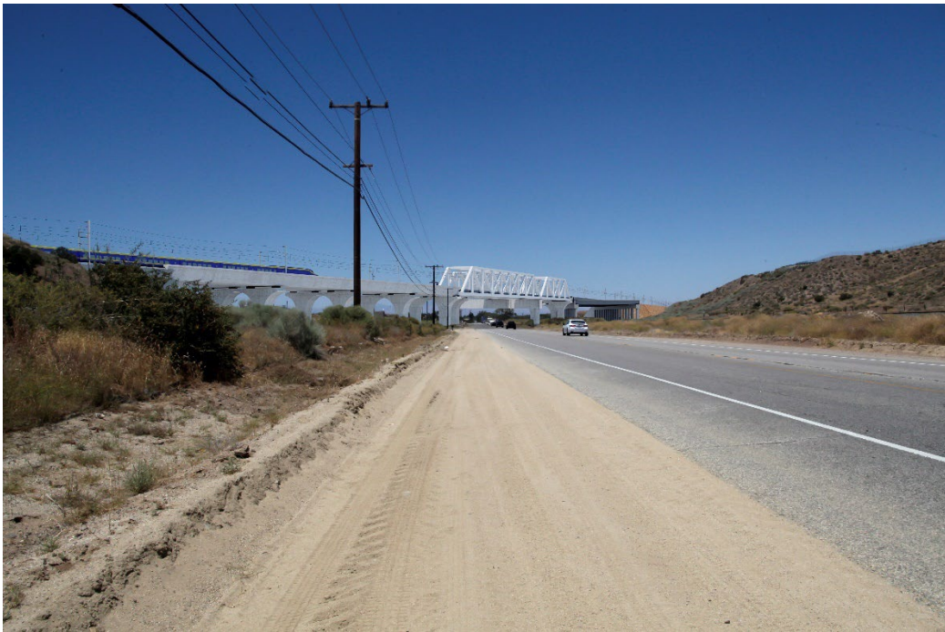
b. Simulated View: The project alignment would cross over Sierra Highway on viaduct. The viaduct would introduce an element of the project environment that would be out of scale with existing visual character, reducing project coherence. The viaduct would be highly visible to motorists and nearby residents blocking distant views and reducing the existing natural harmony. The overall degree of change to visual quality would be adverse.
