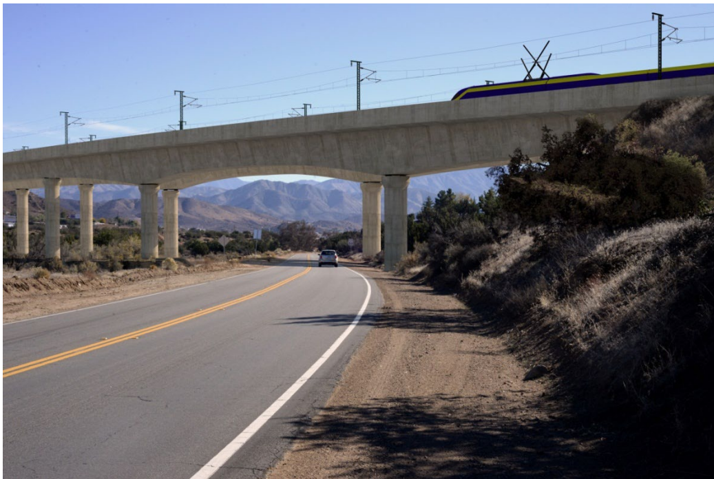
b. Simulated View: The project would introduce a large overcrossing and associated vertical support columns spanning Escondido Canyon Road, that would be out of scale with the existing transportation infrastructure in the setting, reducing the project coherence. The project components would partially obstruct the view of the mountains in the background, reducing the natural harmony at this location; however, this would only be for a short duration for travelers along the road. Overall, the degree of change to visual quality would be adverse.
