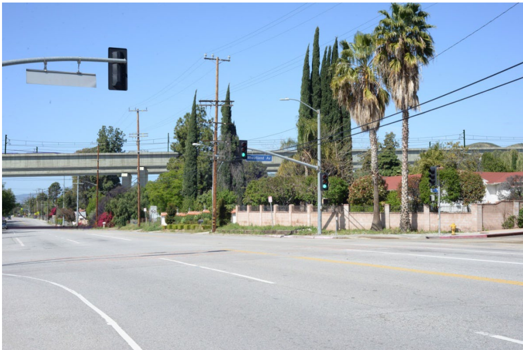
b. Simulated View: The large horizontal scale of the elevated guideway, added by the project, would mirror that of the paved roadway and would also be consistent with the visual character of the nearby overcrossing; it would not change the existing project coherence or cultural order. Overall, the degree of change to visual quality would be neutral.
