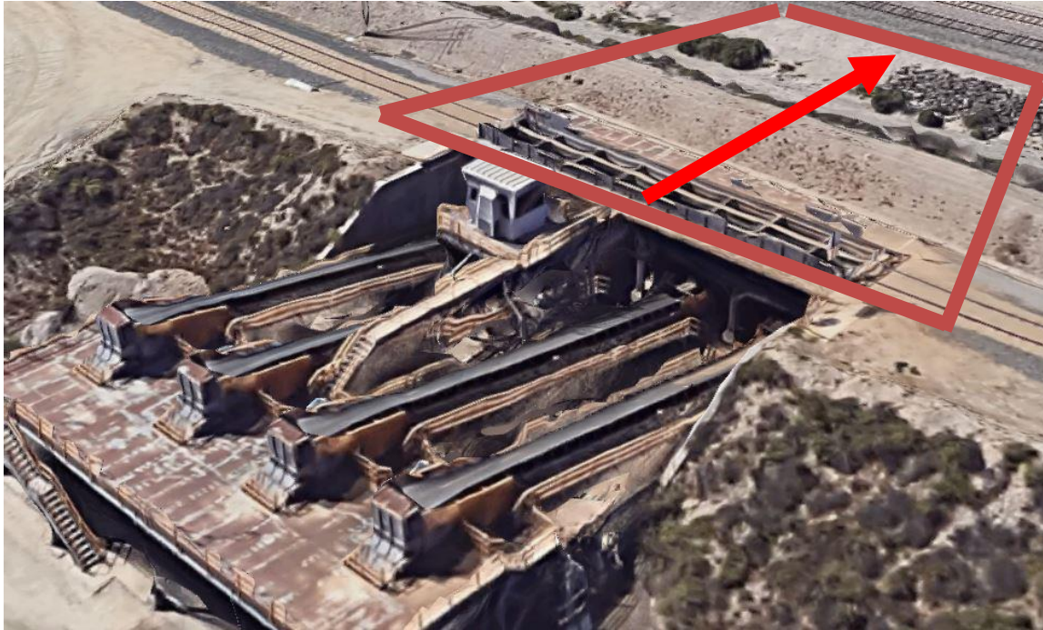
Figure 11-19 Excavation of the New Unloading Pit (Picture of Existing Facility, GE)
