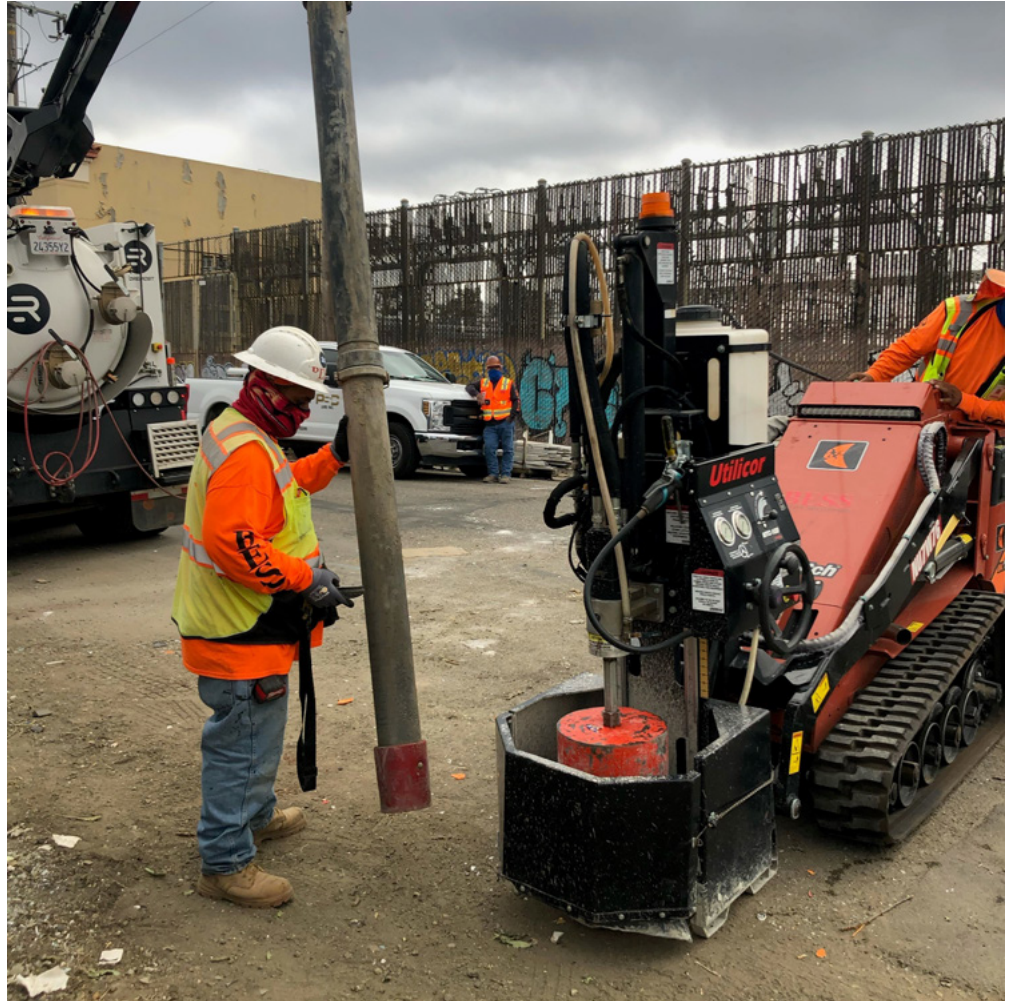
A Bess Utility Solutions crew prepares to drill a hole in the ground using Keyhole technology. The equipment can safely and accurately bore through asphalt and concrete surfaces. The company has been locating, mapping and moving underground utilities for more than 25 years.
