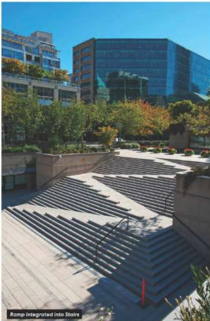
Ramp Integrated into Stairs
