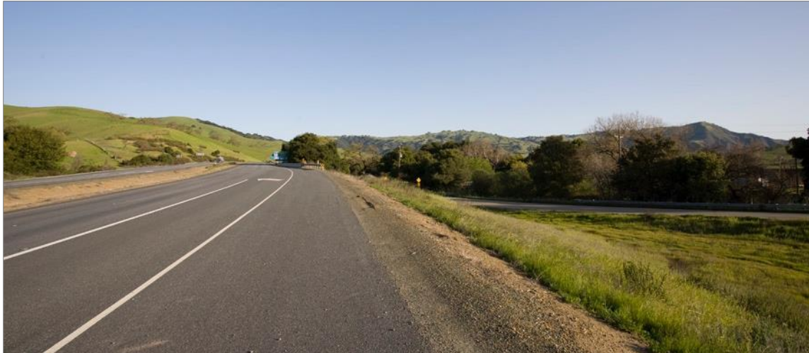
KVP 28—Existing Conditions
