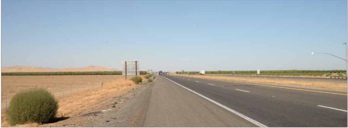
KVP 33—Existing Conditions
