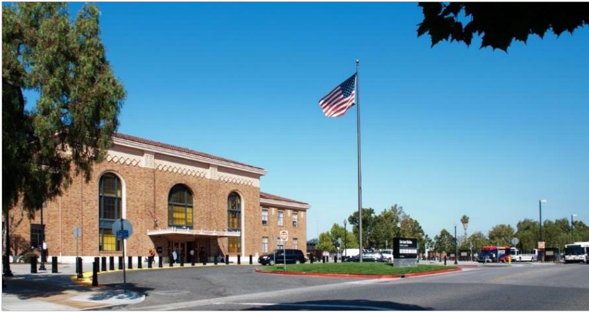
KVP 6—Existing Conditions
