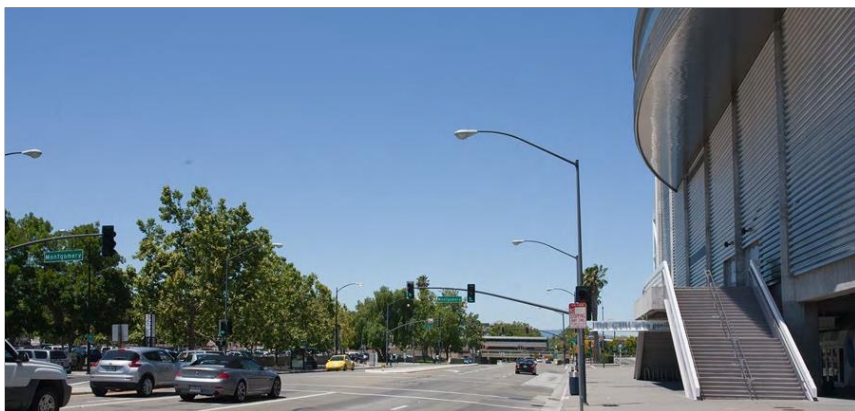
KVP 5—Existing Conditions
