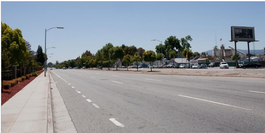
KVP 12—Existing Conditions
