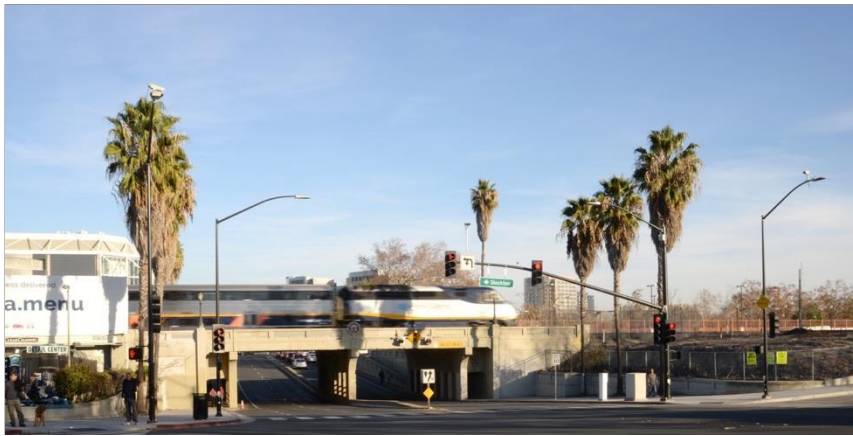
KVP 4—Existing Conditions
