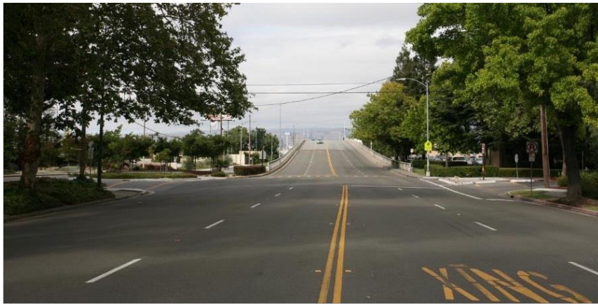
KVP 3—Existing Conditions
