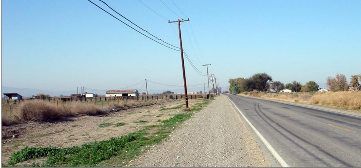
KVP 35—Existing Conditions
