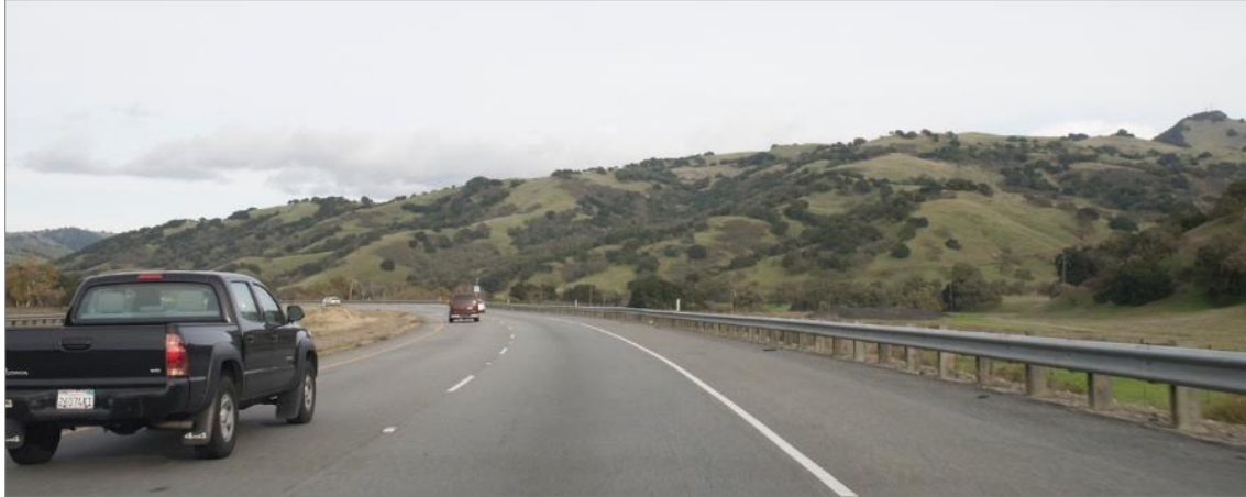
KVP 30—Existing Conditions
