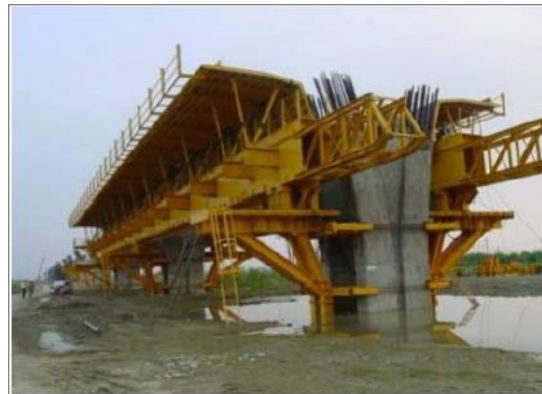
Figure 2-75 Cast-in-Place Construction on Formwork
