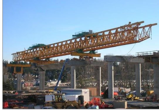
Figure 2-73 Span-by-Span Precast Segmental Construction
