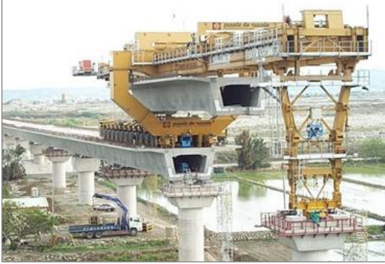
Figure 2-72 Full-Span Precast Construction on Taiwan HSR
