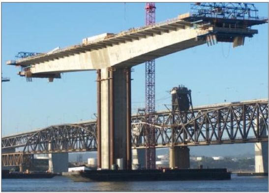
Figure 2-74 Balanced Cantilever Segmental Construction
