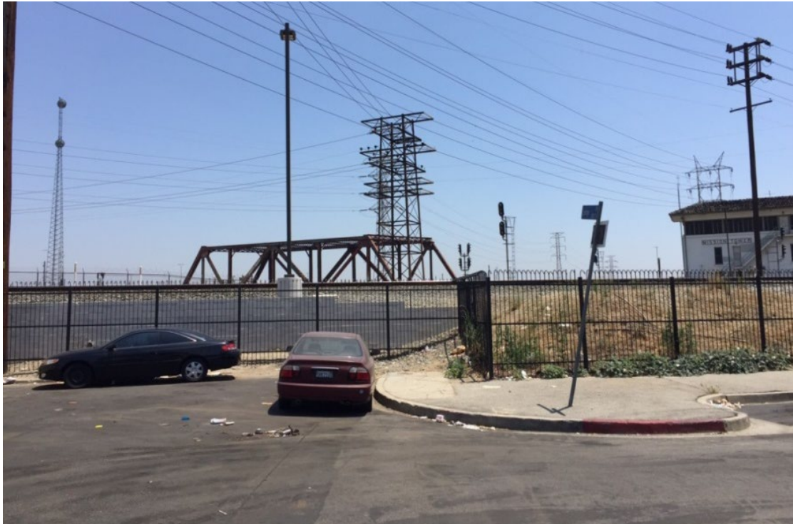
Existing view from Leroy Street in the city of Los Angeles, looking southeast.
