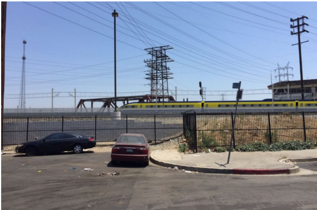
Simulated view of the High-Speed Rail Build Alternative from Leroy Street in the city of Los Angeles, looking southeast.
