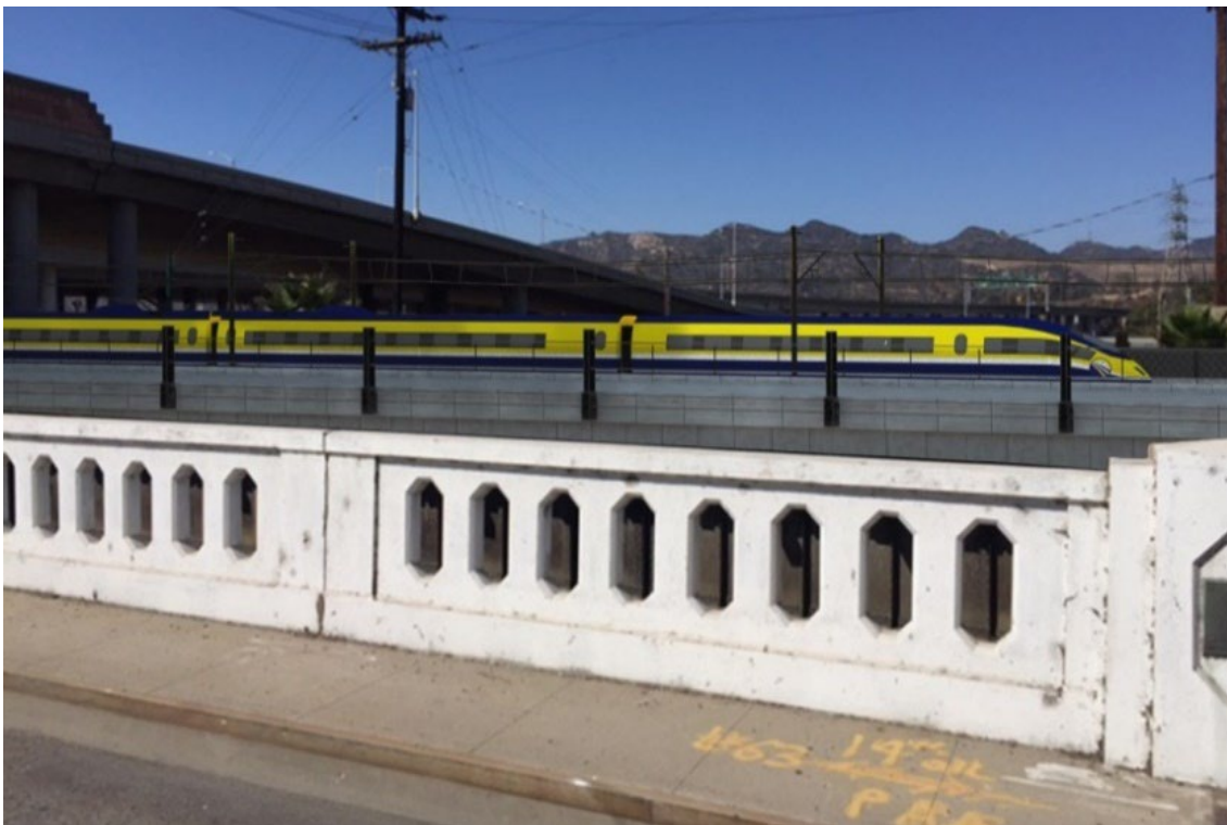
Simulated view of the High-Speed Rail Build Alternative from San Fernando Road in the city of Glendale, looking southwest.
