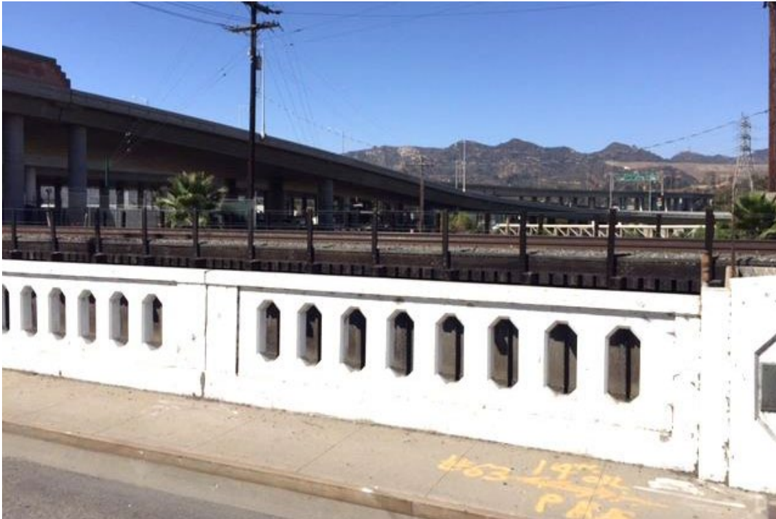
Existing view from San Fernando Road in the city of Glendale, looking southwest.
