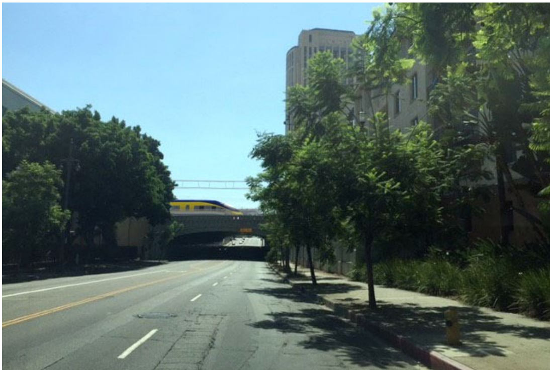
Simulated view of the High-Speed Rail Build Alternative from E Cesar E. Chavez Avenue in the city of Los Angeles, looking southeast.
