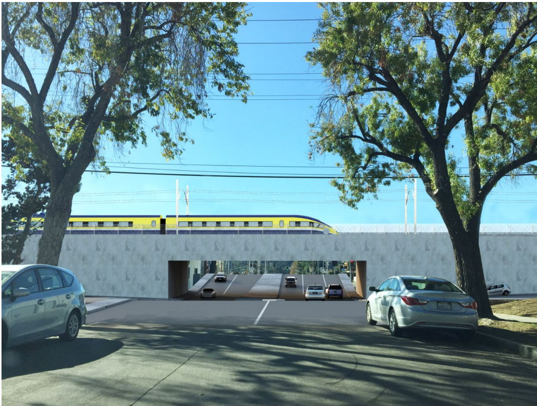
Simulated view of the High-Speed Rail Build Alternative from Pelanconi Avenue/Flower Street in the city of Glendale, looking southwest.
