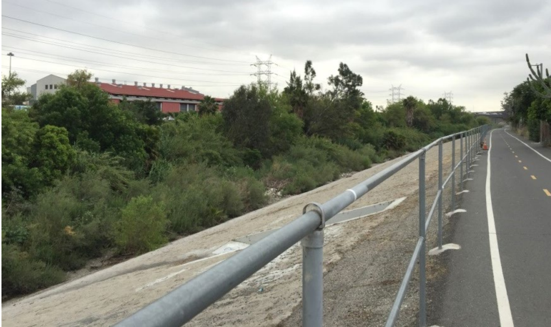
Existing view from the Los Angeles River Bike Path in the city of Los Angeles, looking southeast.
