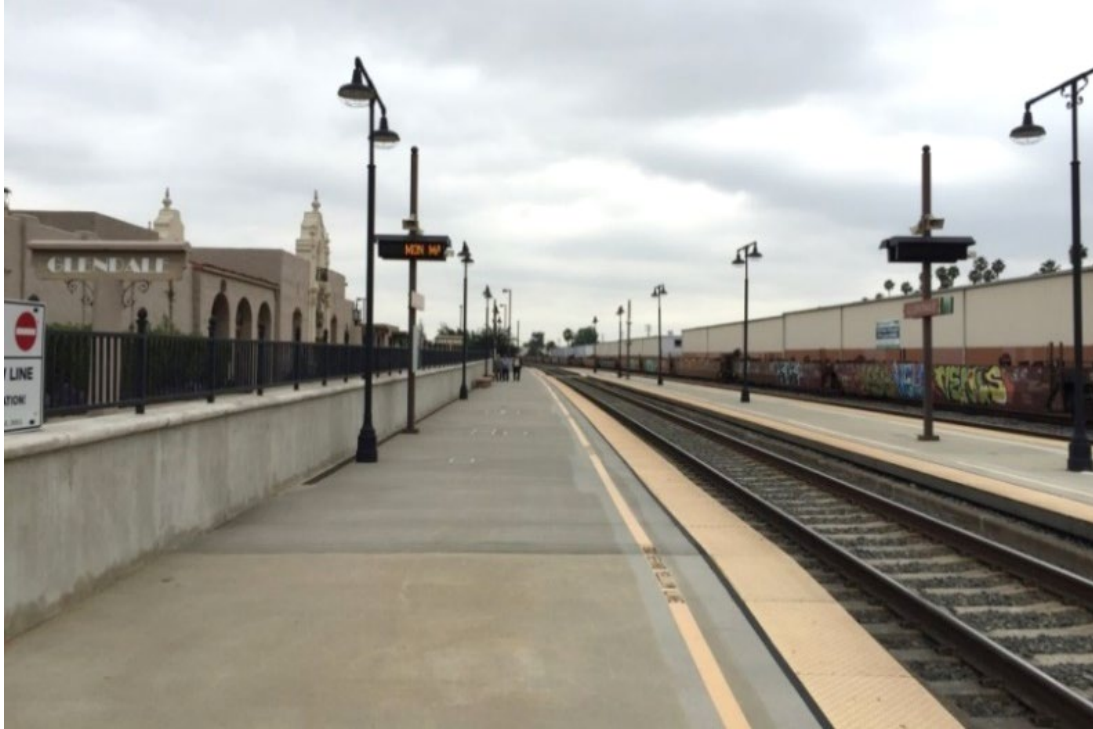
Existing view from the Glendale Transportation Center in the city of Los Angeles, looking southeast.
