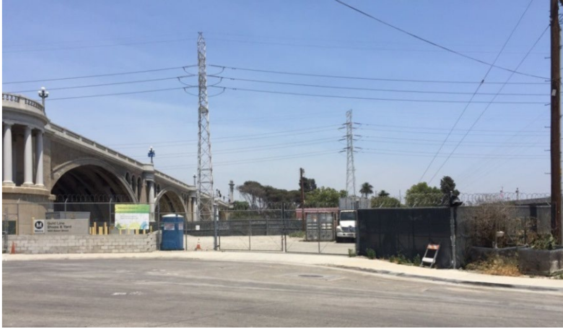
Existing view from Los Angeles State Historic Park in the city of Los Angeles, looking northeast.
