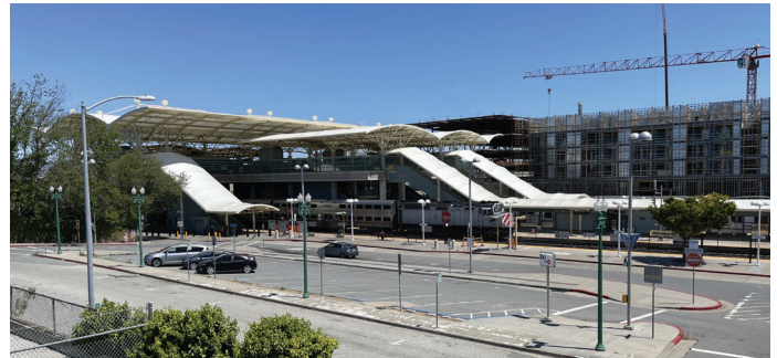
The Millbrae-SFO Station will provide connections from high-speed rail to BART, Caltrain, SamTrans, and other transit providers.
