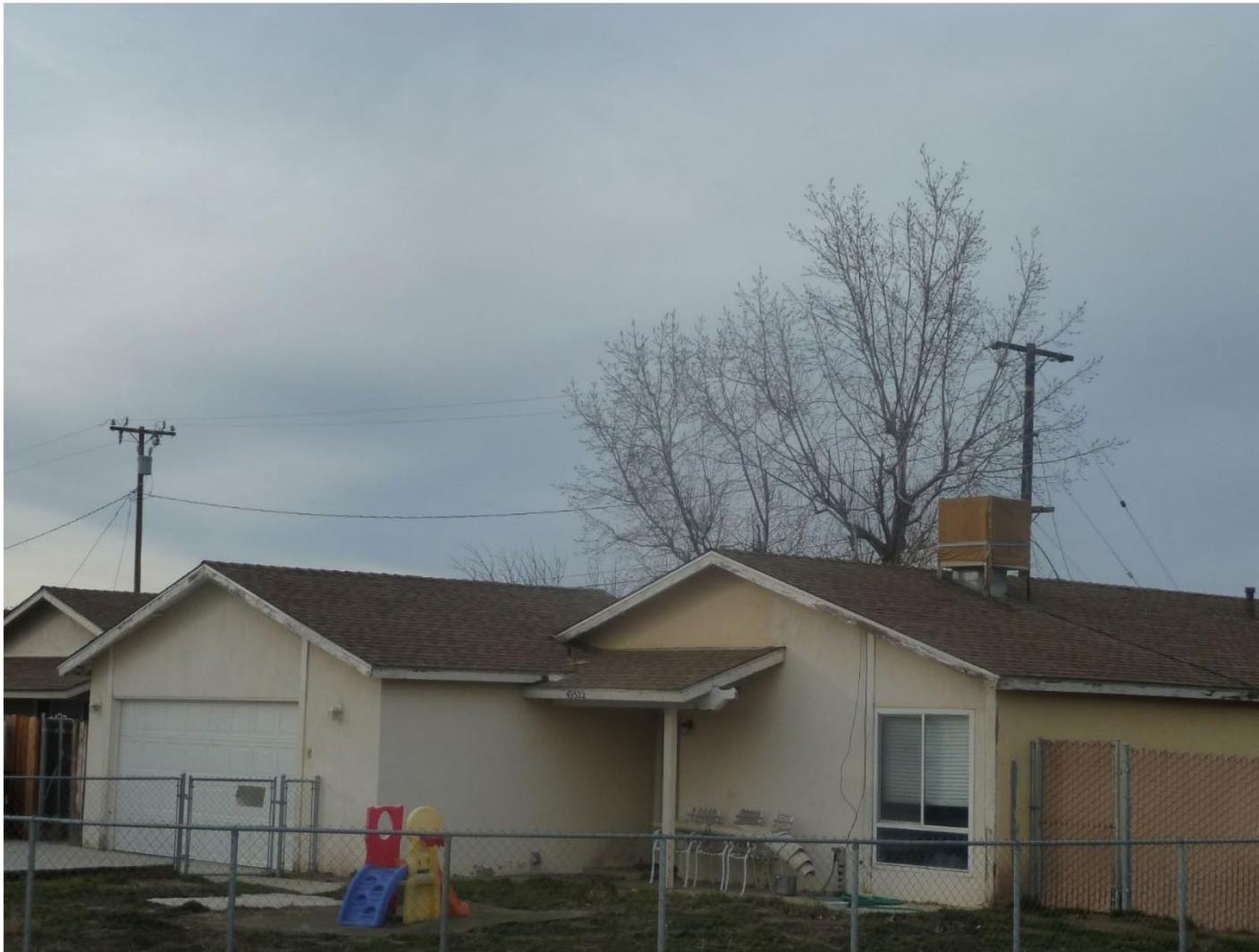
Figure A3.5-5(c) Location 05: Alan Avenue and Lois Street, Tehachapi
