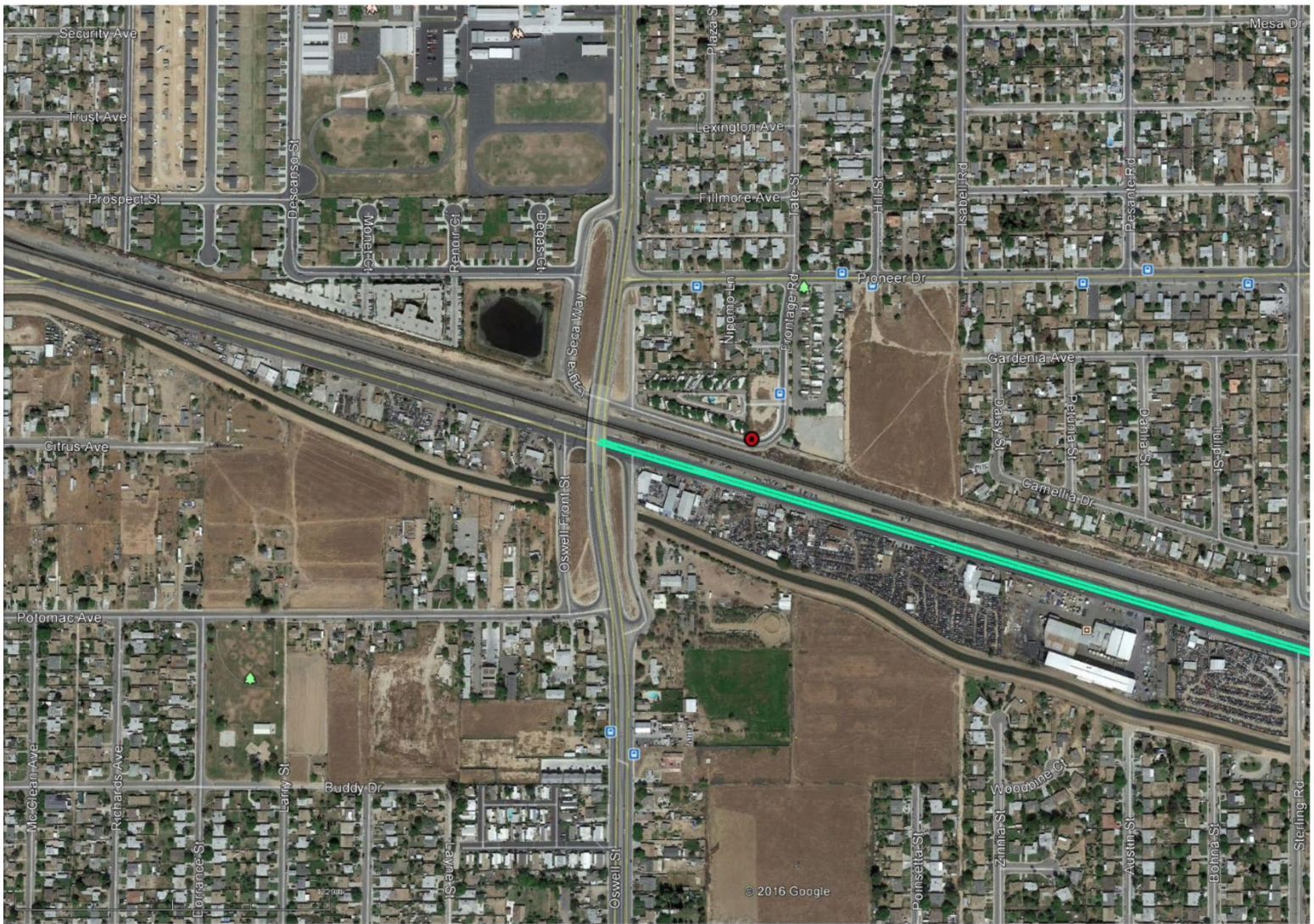
Figure A3.5-1(a) Location 01: Laguna Seca and Oswell Streets, Bakersfield Urban setting adjacent to the existing UPRR alignment, with significant RF emitters (Lat 35° 22' 00.99", Lon W118° 56' 53.05")
