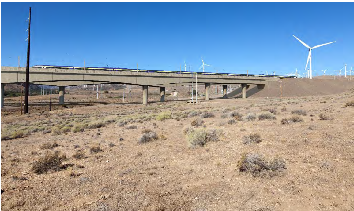
Figure 3.16-36 Key Viewpoint 18a: Existing and Simulated Views of Alternative 1 from the Existing Alignment of the Pacific Crest Trail Looking West
