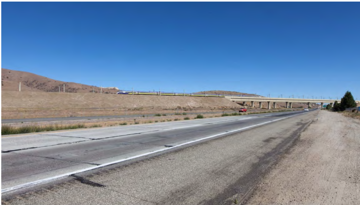
Figure 3.16-33 Key Viewpoint 15: Existing and Simulated Views of Alternative 1 from State Route 58 Looking Southeast
