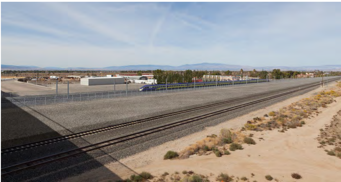
Figure 3.16-42 Key Viewpoint 25: Existing and Simulated Views of Alternative 1 from Avenue L Overpass Looking Northwest
