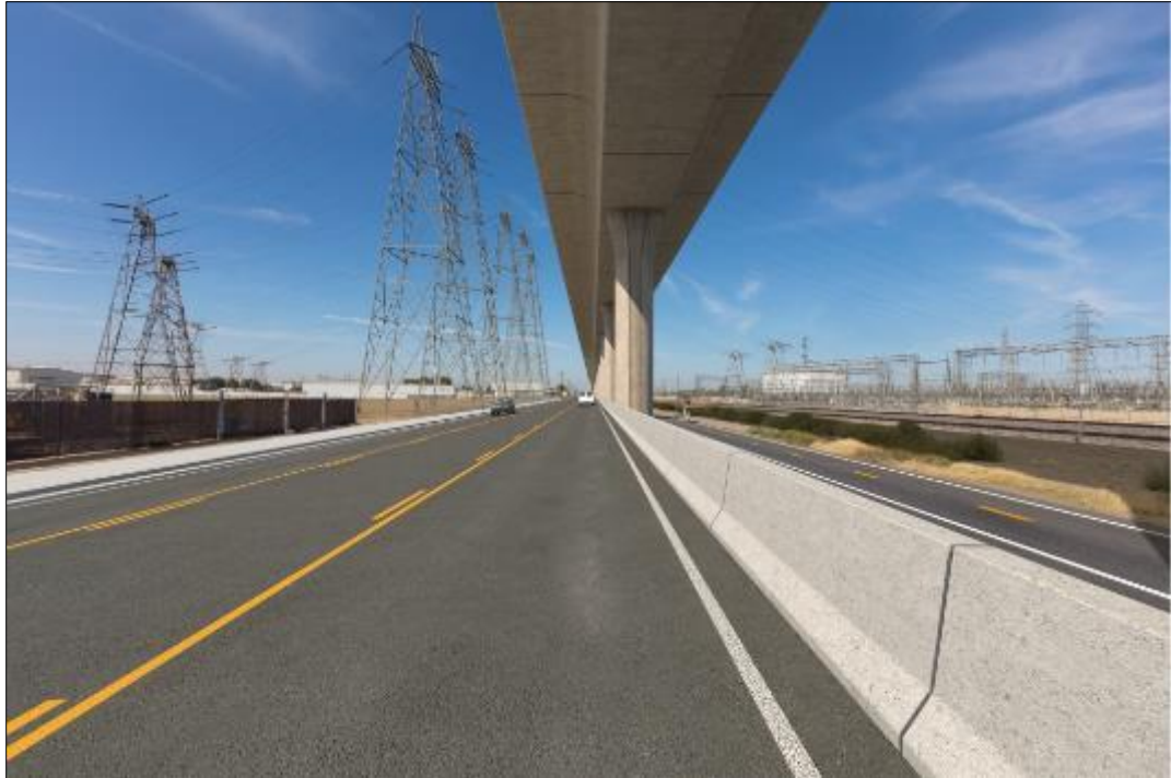
Figure 4-6 Magunden Substation, Proposed Design—Option B. The VERs would relocate the existing towers at left further south to make space for a traction power station.
