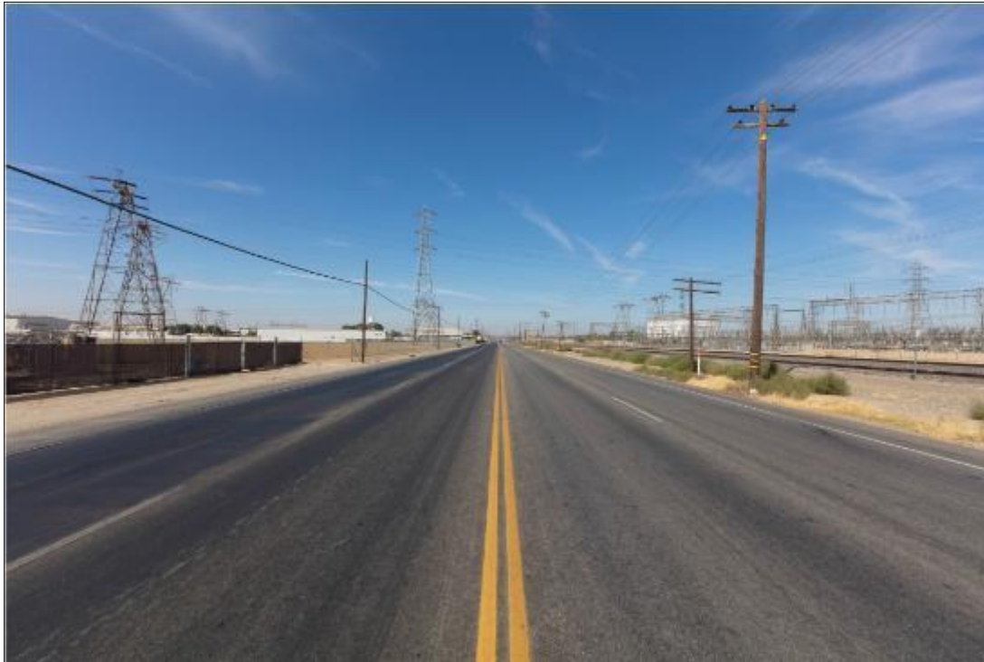
Figure 4-4 Magunden Substation Vicinity, Existing Site—Camera Facing West
