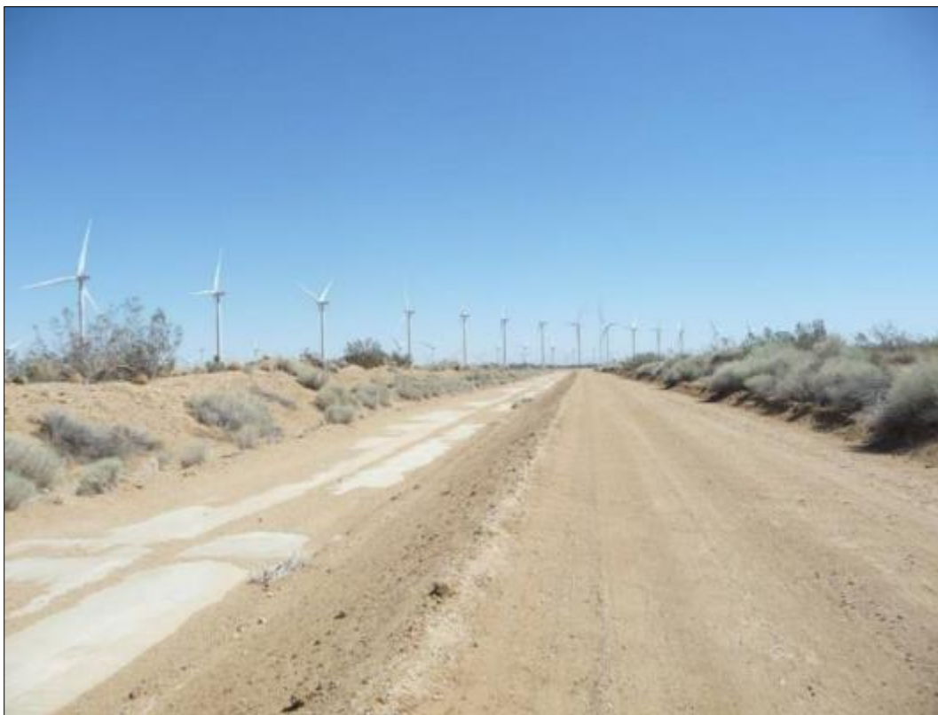
Figure 4-8 Los Angeles Aqueduct, Typical Segment West of Rosamond
