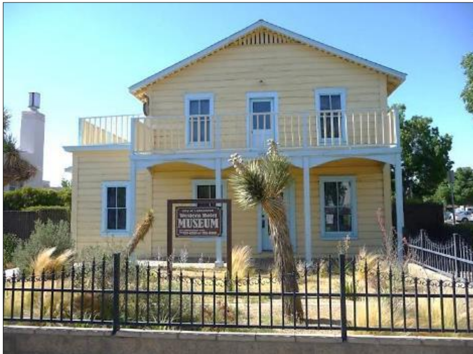
Figure 4-15 Western Hotel, 557 W Lancaster Boulevard, Lancaster
