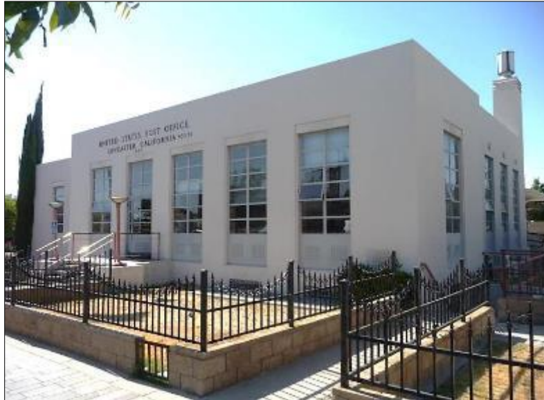
Figure 4-11 Lancaster Post Office, 567 W Lancaster Boulevard, Lancaster
