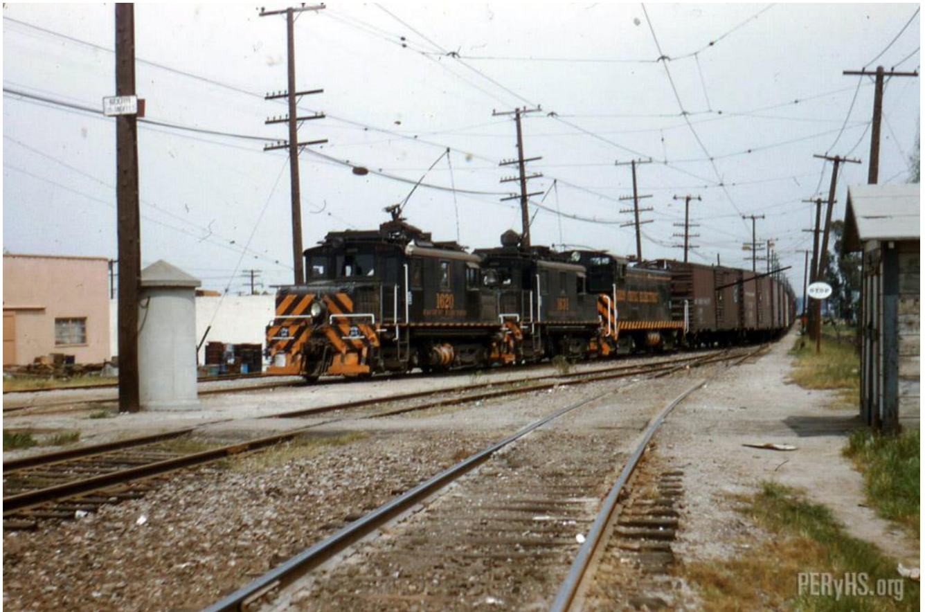
Electric freight trains were once common in Southern California: Pacific Electric Railway all-electric local freight train in South LA, 1953 (Photo: Pacific Electric Railway Historical Society)
